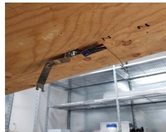
Mounting bracket fastened to ceiling
